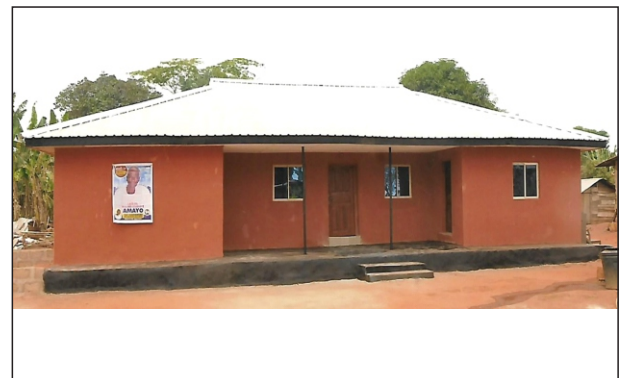
HOUSE OF THE ODIONWERE OF ODIGUETUE COMMUNITY, OVIA NORTH EAST LGA, RENOVATED BY OOPC
