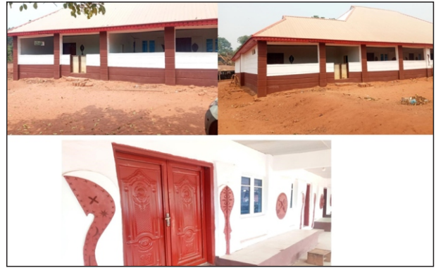
PALACE OF THE ENOGIE OF UMOKPE, UHUNMWONDE LGA, RENOVATED BY OOPC
