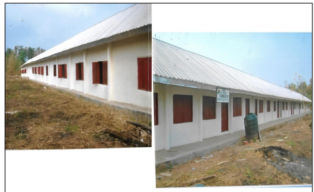
FIRST PHASE OF THE CONSTRUCTION OF IDIA SECONDARY SCHOOL, OKE COMMUNITY, UHUNMWONDE LGA
